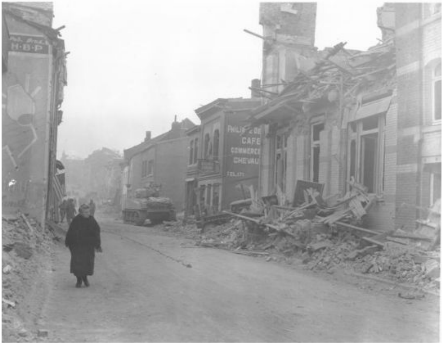
Damage to the city of Bastogne, Belgium on December 26, 1944
